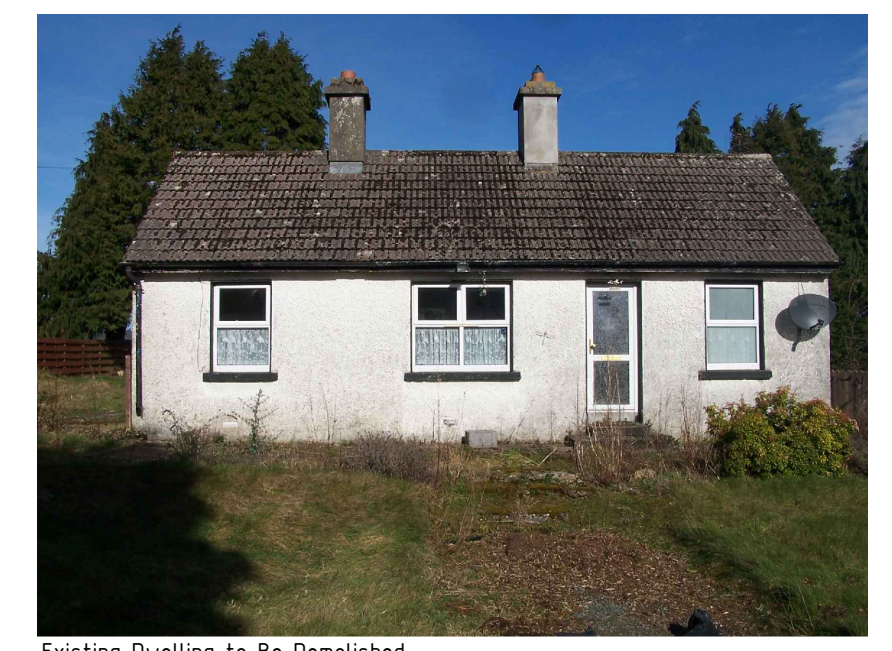
Existing Dwelling to Be Demolished.
